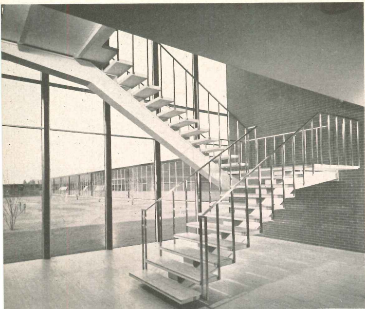
Service Administration Building Stair
