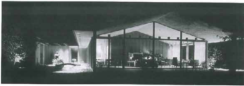
Van Meter Residence Springfield, Illinois, 1962-63 Architects: King & Murphy
