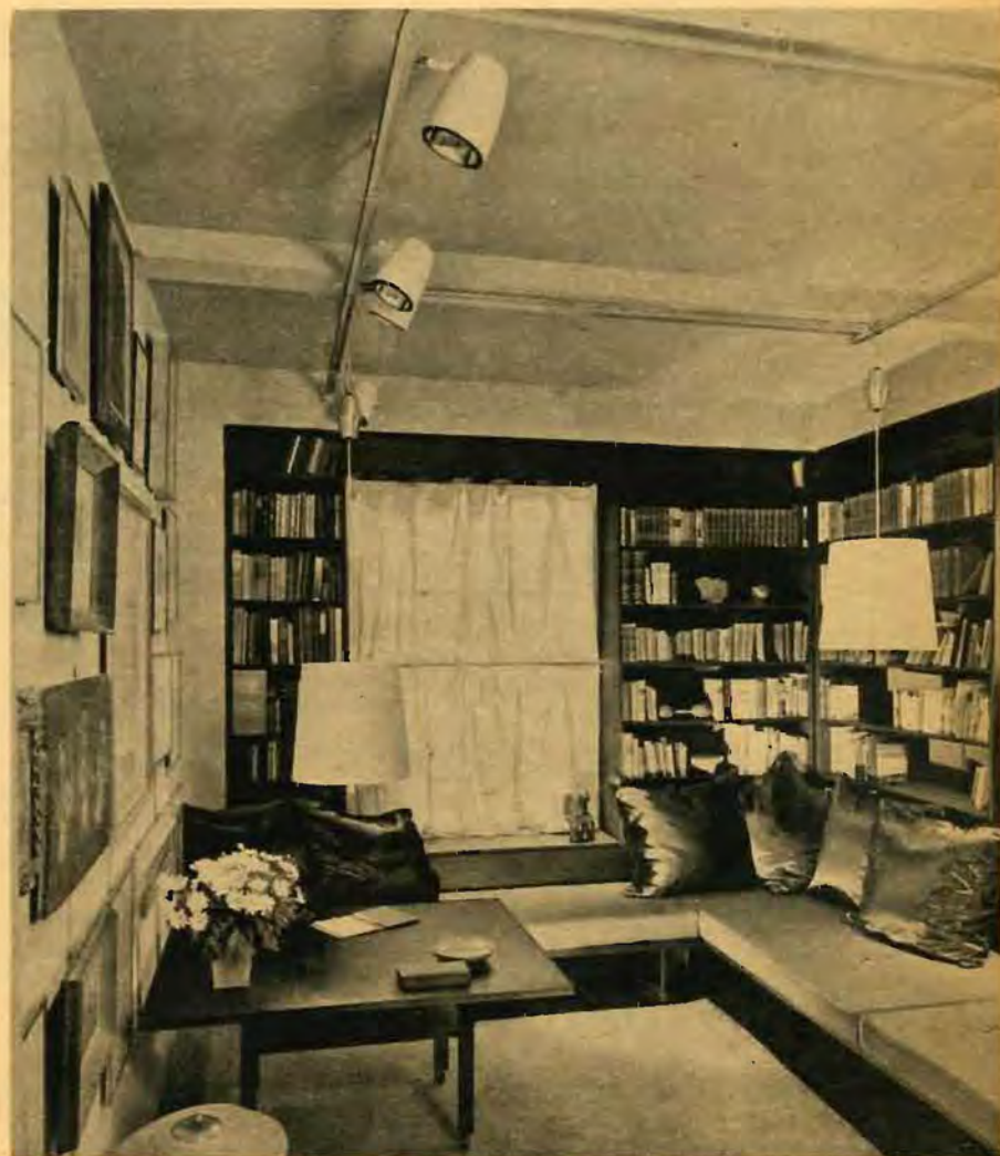
CEILING FIXTURES in the library take the place of portable reading lamps and also illuminate the pictures. Installation consists of four Lightolier electrified aluminum poles screwed to the ceiling to form an open square, and fitted with shaded lamps for reading and spotlights for the pictures. The adjustable hanging lamps can be raised, lowered, and like the "spots," moved along the poles to suit the individual's convenience. Fixtures, Marie Nichols.
